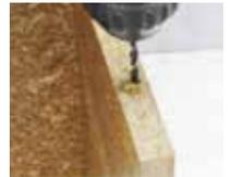
To ensure that the panel edge does not split, the spacing between nails should not be less than 100mm. And the distance from a nail to the panel edge should not be less than 70mm.
